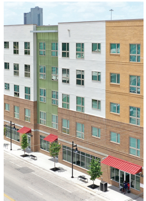
MULTI-FAMILY COMPLEX Fort Worth, Texas
