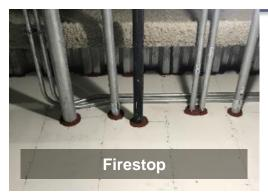
Firestop is passive protection that impedes the passage of fire, smoke, and gases in a fire-rated floor or wall
